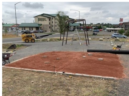
Photos: Boothill Sign Relocation Project
