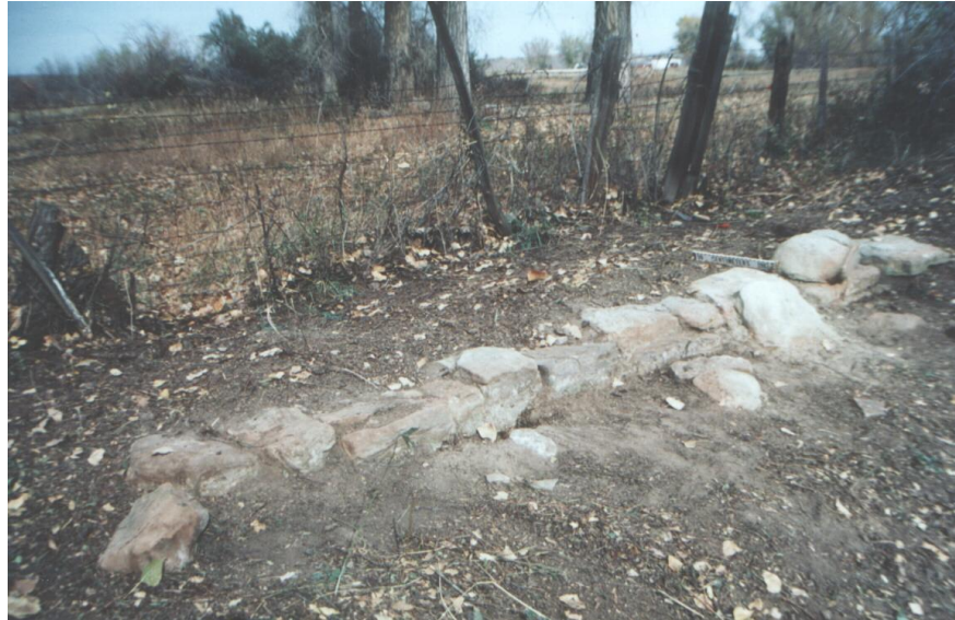
Picture # 1: This photo shows Tracy's Dock (24YL1209) after the duff is brushed off. This image was taken on 10/17/87 as part of the Tracy's Landing project for the Montana State Historical Preservation Office.
