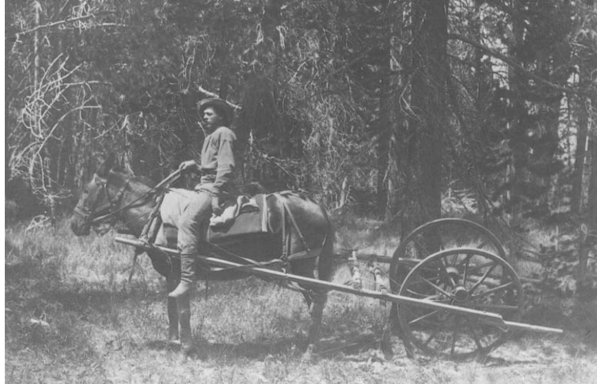
This photo shows a 19 th century odometer. This type of instrument was used by the military expedition on the Yellowstone in the summer of 1872. Dept. of the Interior, National Park Service, Yellowstone National Park
